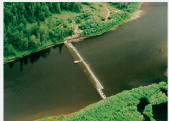
An aerial view of the Takotna River weir (credit all weir photos: Kevin Whitworth).
